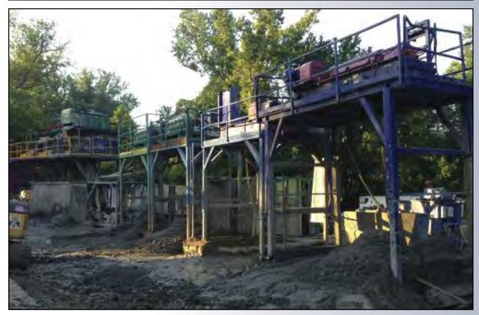
The ground needs to be excavated, transported, and separated for the slurry-based microtunneling system to work.
