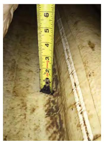
Trapped Water from Potential Infiltration in CIPP Liner
