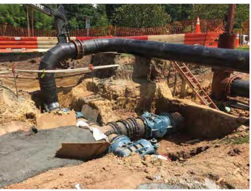
24-inch Tee and Plug Valves Installed Downstream of Line Stop
