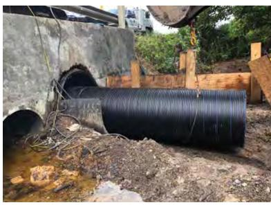
The DuroMaxx SRPE Liner Pipe offered a fully structural reline solution
