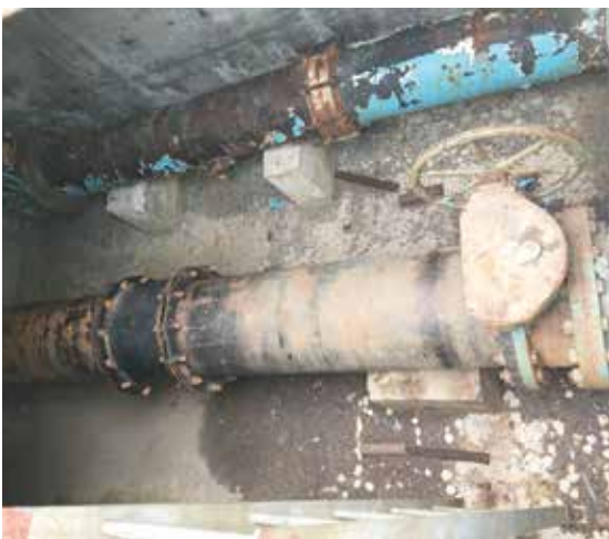
Abandoned Meter Vault used for Insertion
