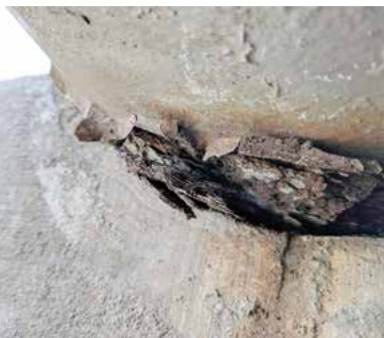
Close up of Pipe Support (59% wall loss)
