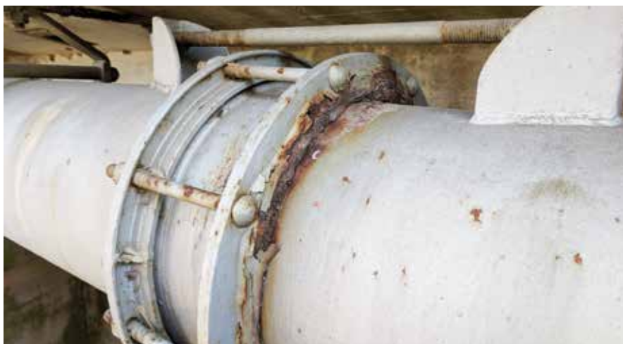
Corrosion at Mechanical Coupling
