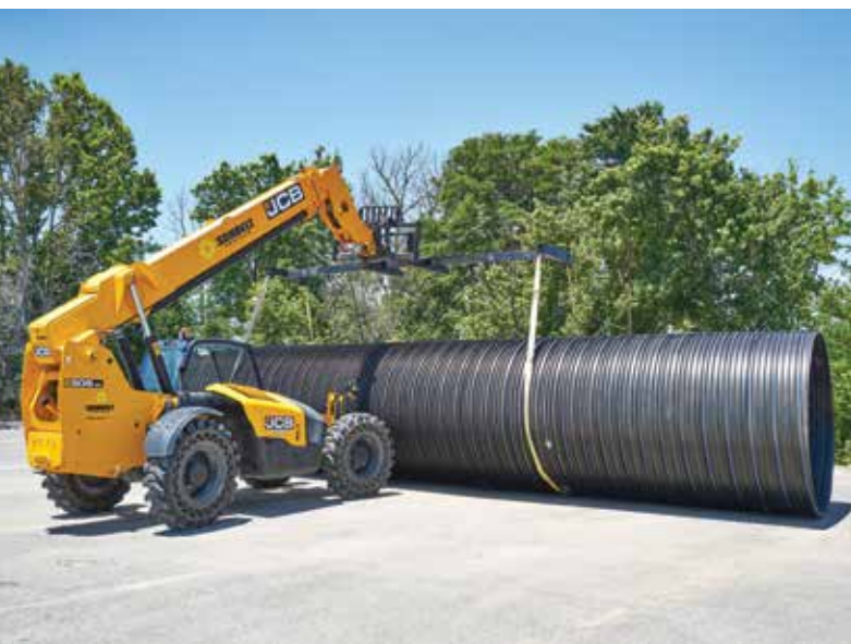
Liner pipe was shipped directly to the site in 41-foot and 45-foot sections
