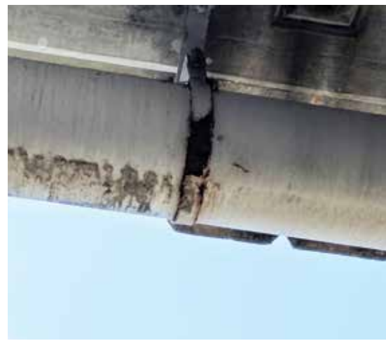
Localized Wall Loss at Pipe Hanger
