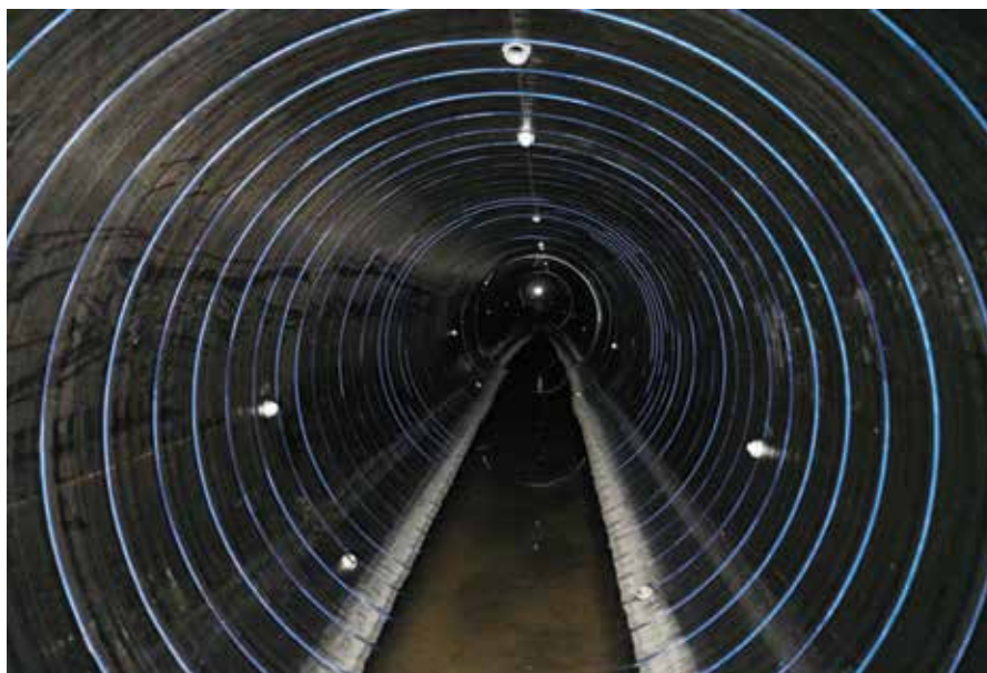
The DuroMaxx SRPE Liner Pipe offered a fully structural reline solution
