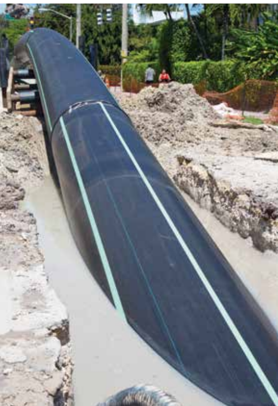
Fused HDPE pipe entering the pit. More than 4,200 feet of 54-inch diameter HDPE PE 4710 pipe was used
