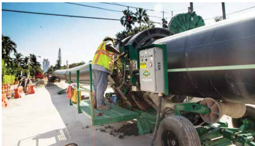
An ISCO field tech used a McElroy 2065 fusion machine to make the final tie in
