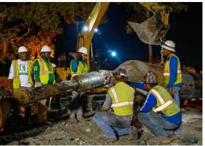
DMSI and Centerline staff inspect the connection between the reamer and pipe string prior to pullback
