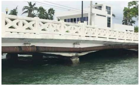
Existing water main aerial crossing showing significant joint deflection, pipe corrosion, and pipe support failures
