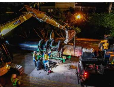
Butt fusion of the pulling head onto 36-inch HDPE piping
