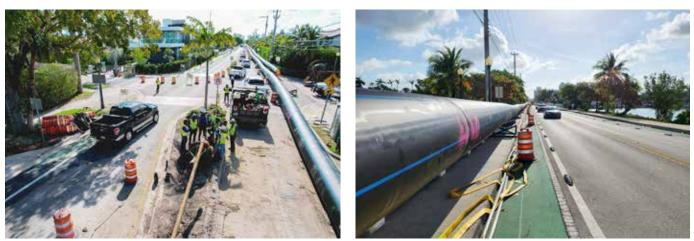
MOT plans allowed for flagged two-way traffic when pipe was fused and strung out for pullback along the two-lane road
