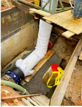
The resin-impregnated tube inverts and travels the length of the host pipe
