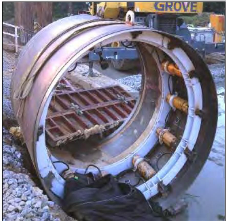
*Bradshaw provided intermediate jacking stations and a high-volume bentonite lubrication pump.*
