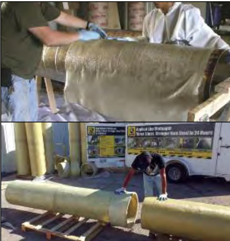
Figure 2. StifPipe is made and connected on site.
