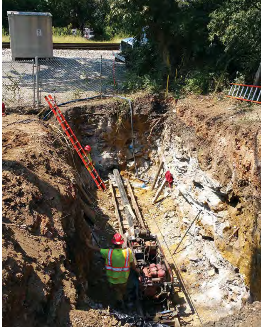
The crossing under the railroad easement was through 120LF hard limestone
