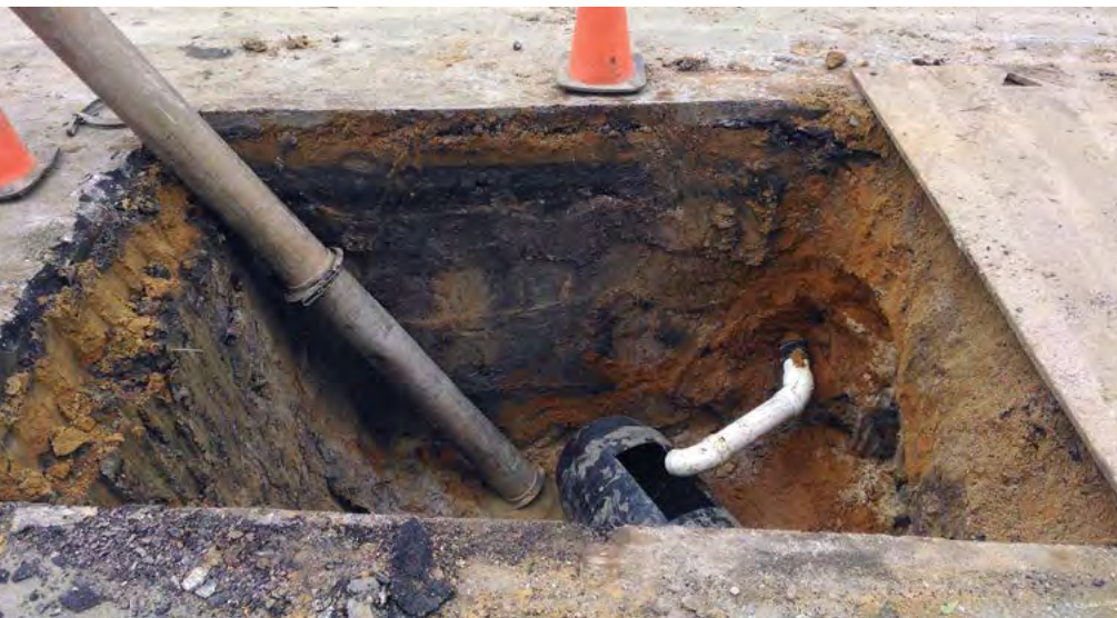
Maintaining service to residential laterals
