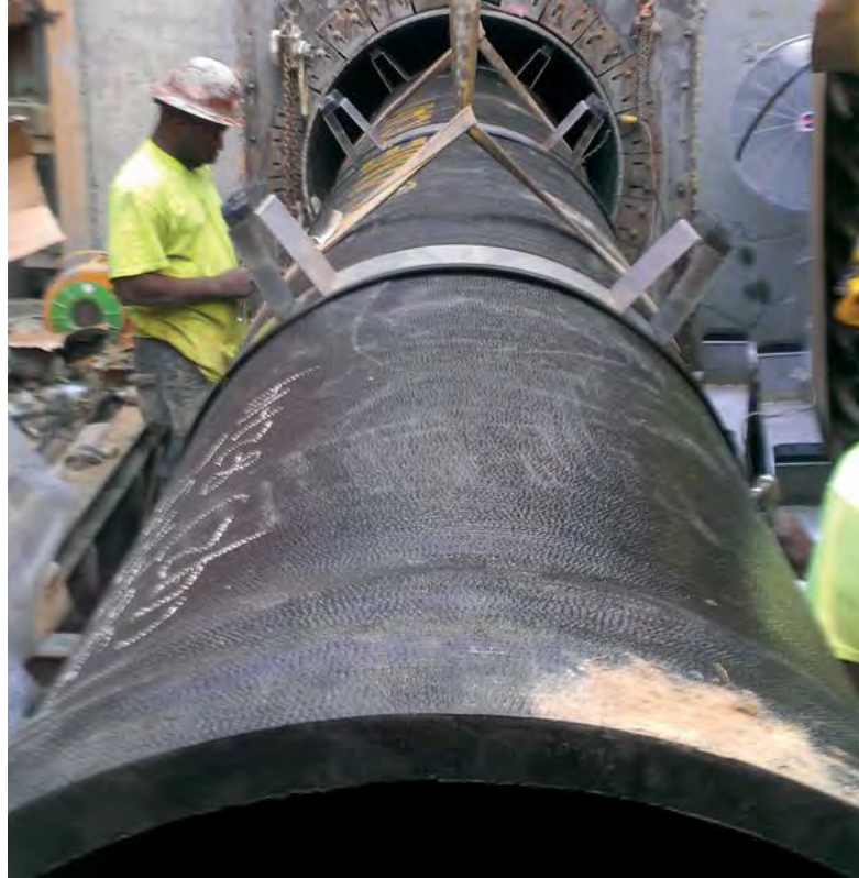
DIP carrier pipe readied for installation with casing spacers in place
