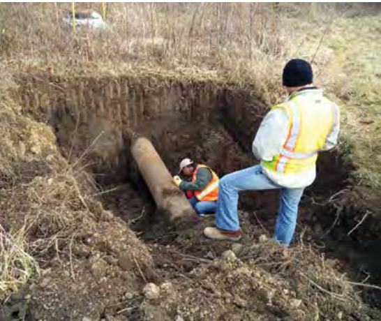
Excavated Pit for Ultra Sonic Testing
