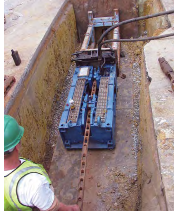
Pipe bursting machine pit
