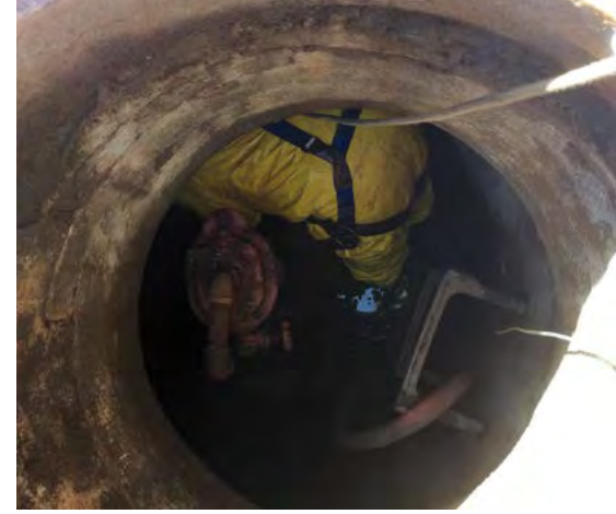
Testing in ARV Manhole
