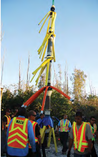
Crews prepare inspection tool for deployment.
