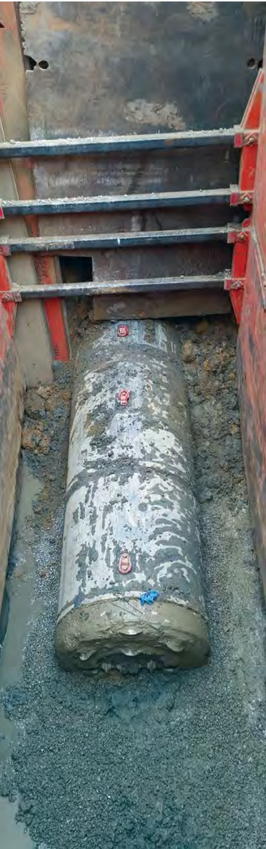
MTBM recovery in receiving shaft
