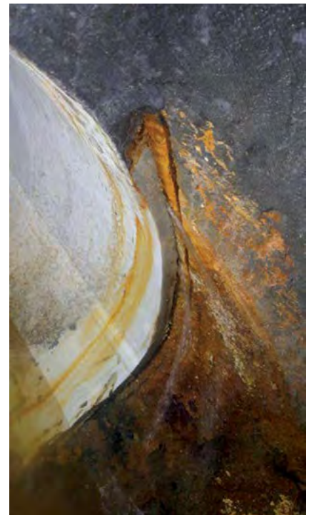
Infiltration between the host pipe (54 inch Diameter) and the new CIPP liner.
