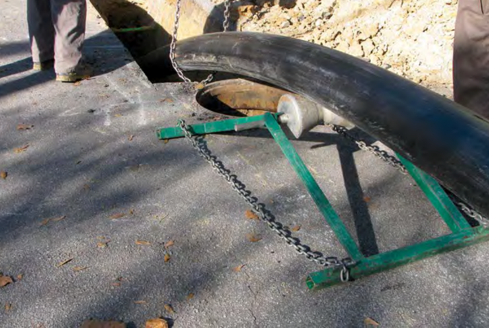
Pipe insertion pit
