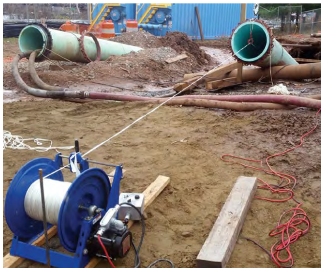
The Accurate Mapping Probe was also utilized to verify pipe location and bend radius of HDD pipe after another installation.
