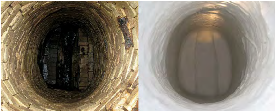
CIPM™ liners form a complete reinforced structure within the host structure and are easily installed
