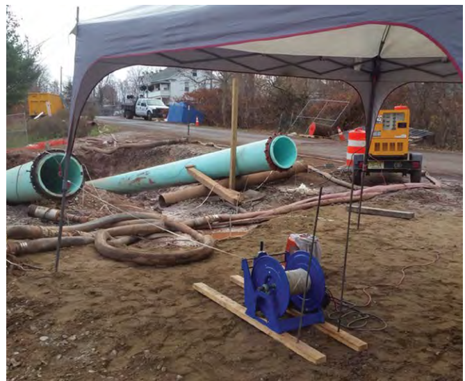
The Accurate Mapping Probe was also utilized to verify pipe location and bend radius of HDD pipe after another installation.
