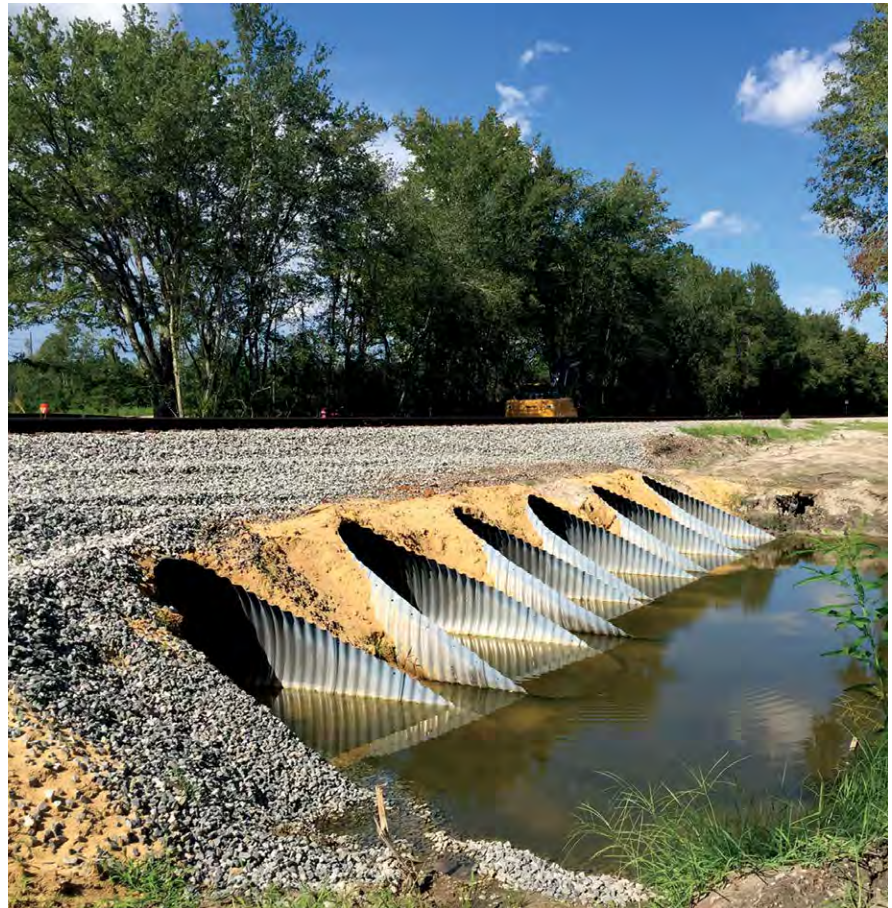
Grouting and backfilling the area reduced ongoing maintenance costs.
