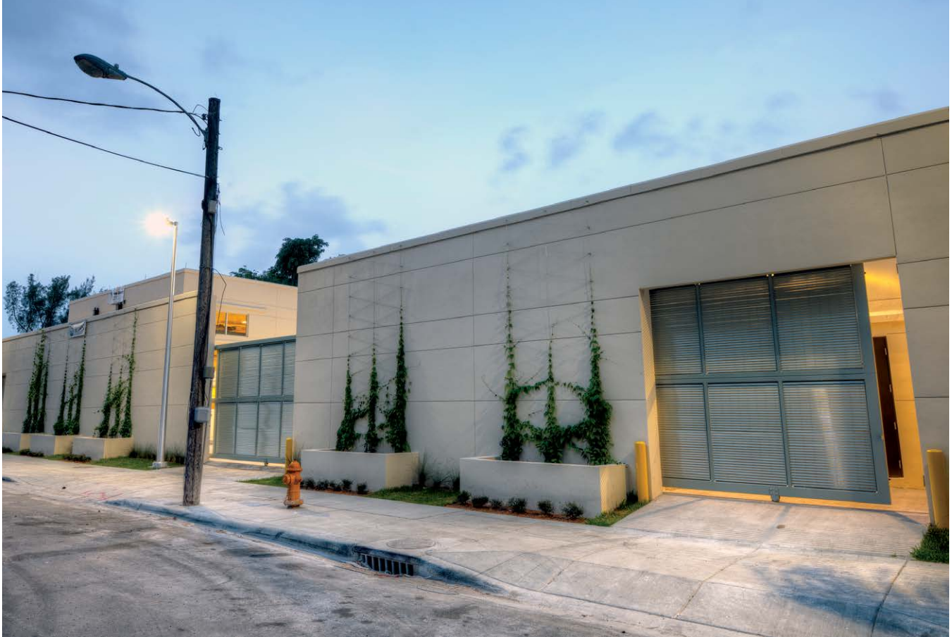
MWH designed the pump station to be aesthetically pleasing and fit in with the local community
