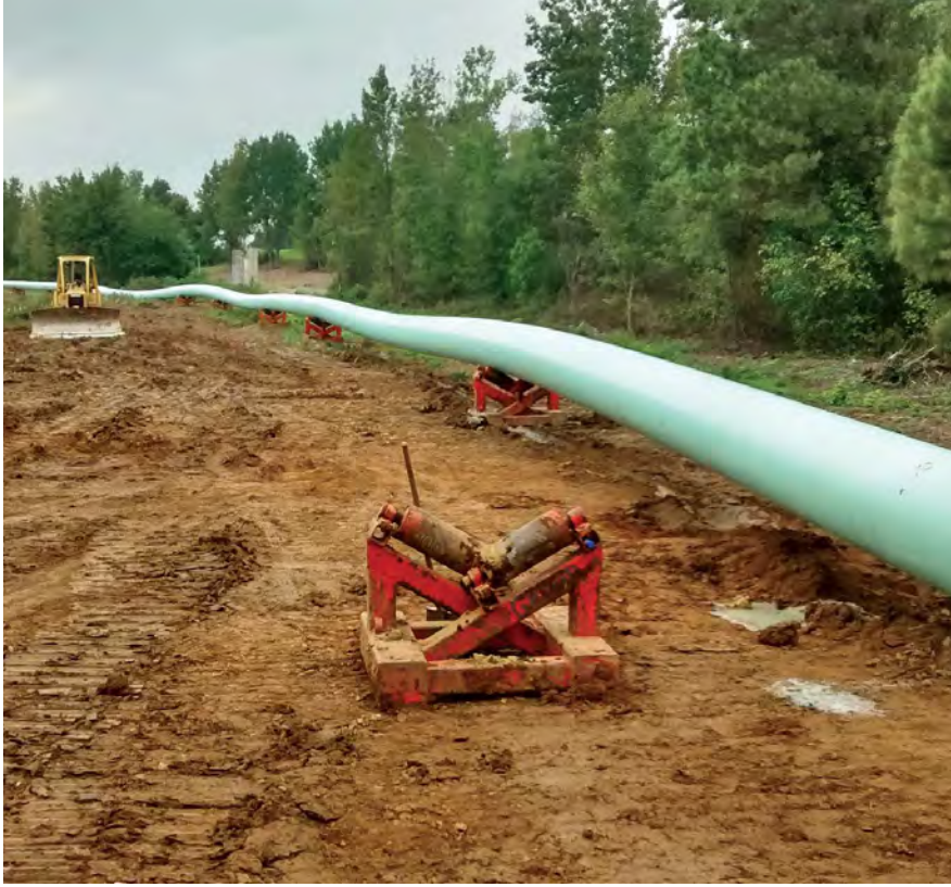
Figure 2. fPVC Pipe String
