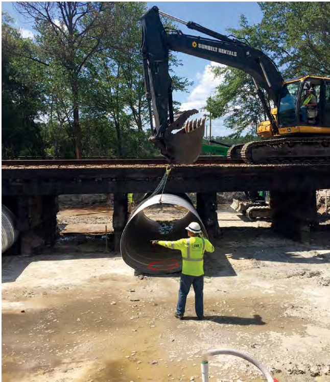
CSX track workers dewatered the area and placed the CSP segments
