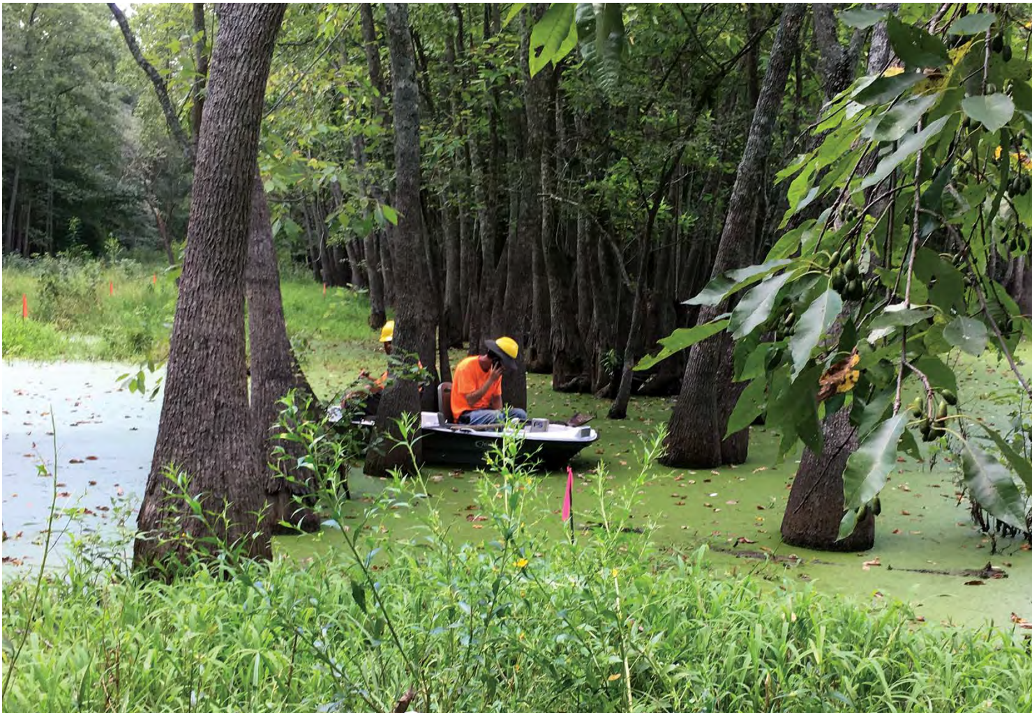
Figure 3. Pilot Bore Tracking Boats
