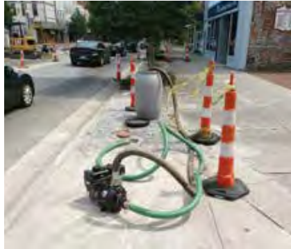
Maintaining service to businesses along Queen Street
