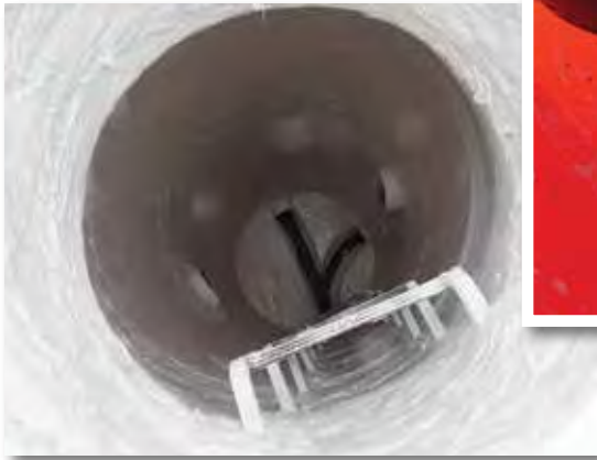
Re-lined Manhole on Wankinco Avenue
