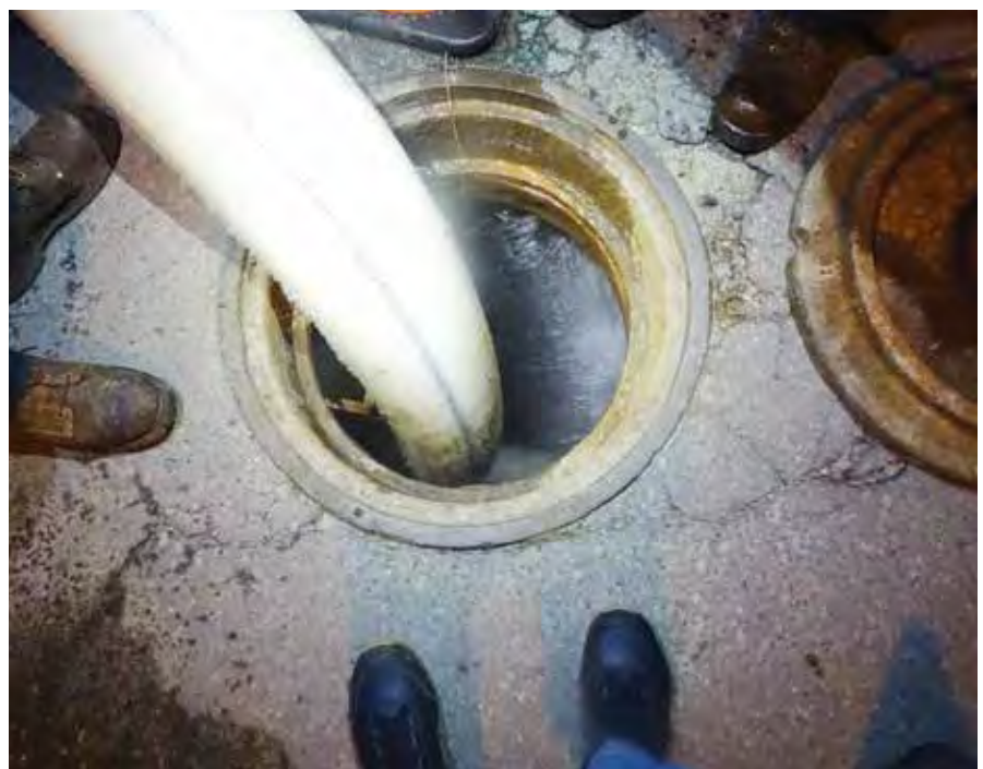
Liner inversion and curing worked very well at pipe deflection
