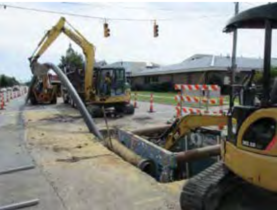
Pipe bursting pipe insertion pit in the center of Queen Street
