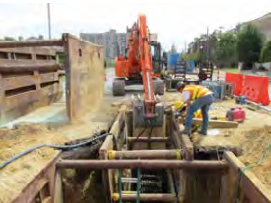
Pipe bursting machine pit in the center of Queen Street
