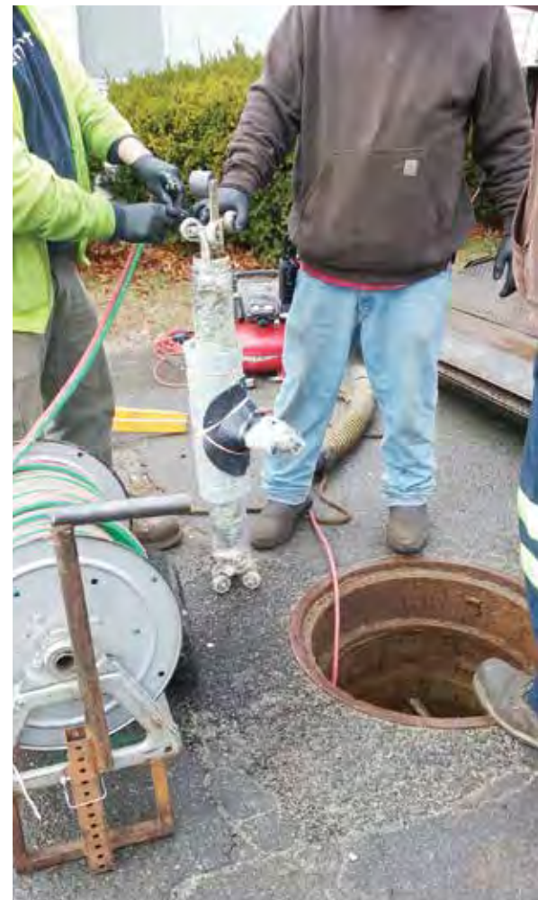
Tee Liner with inflatable packer assembled and ready for insertion
