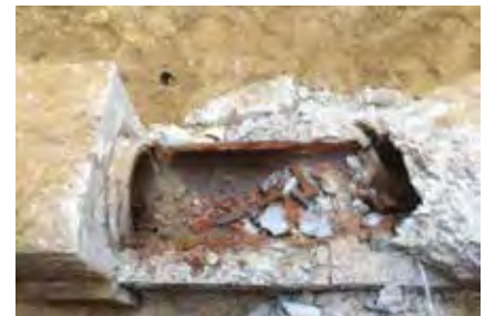
Concrete encasement around 15-inch clay sewer
