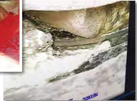
Rock in pipe near area of deflection. A very challenging job
