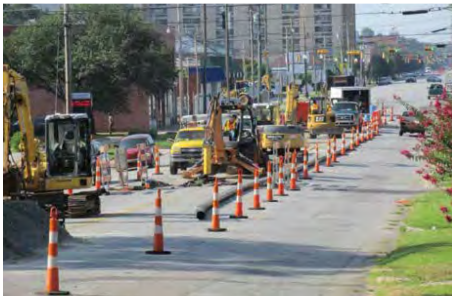
Pipe bursting down the center of Queen Street, Kinston, NC
