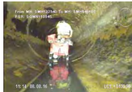
Tool Cart with Emergency Oxygen, Handheld Laser, Sounding and Probing Equipment
