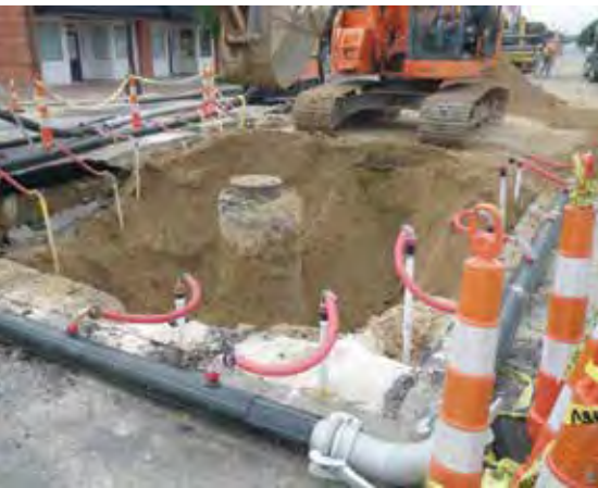
Well pointing for deep excavations in Queen Street
