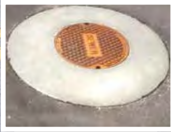
A circular cut core removes potential concentrated stresses and has many other advantages
