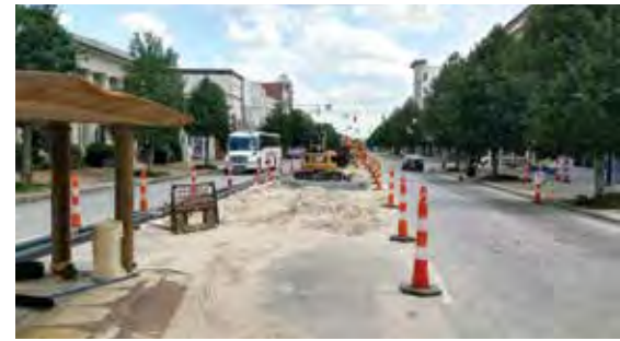
Installing service laterals along Queen Street
