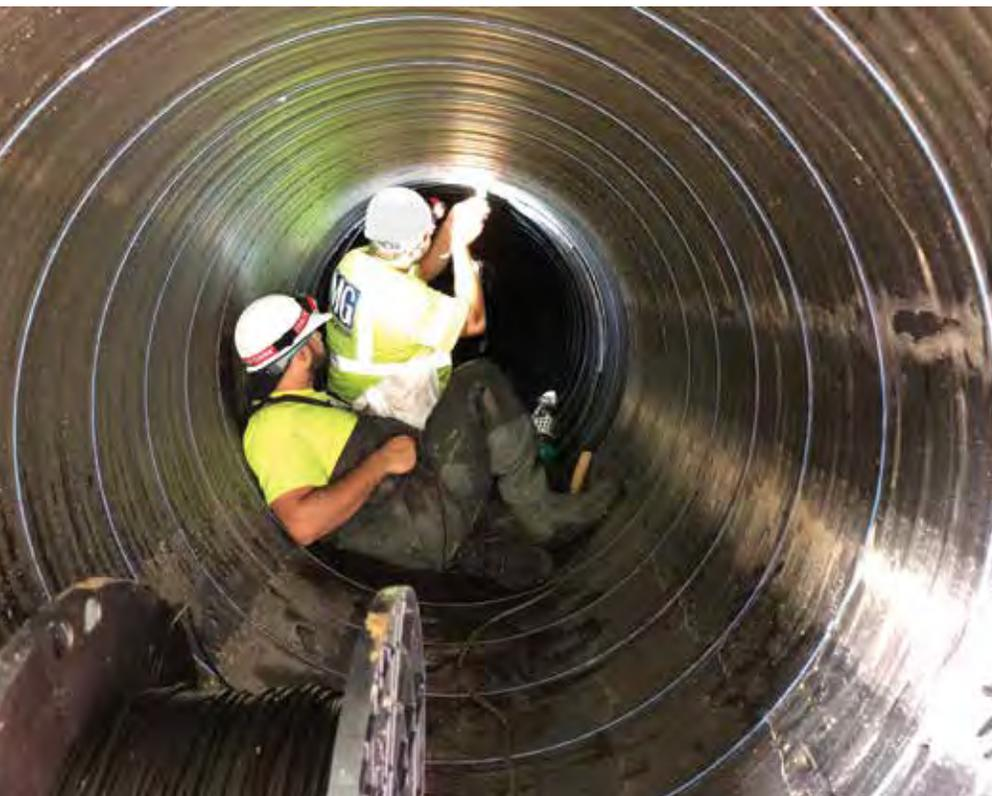
*Welded Coupler (WC) joints were included in the design to provide a 30 psi, watertight joint*
