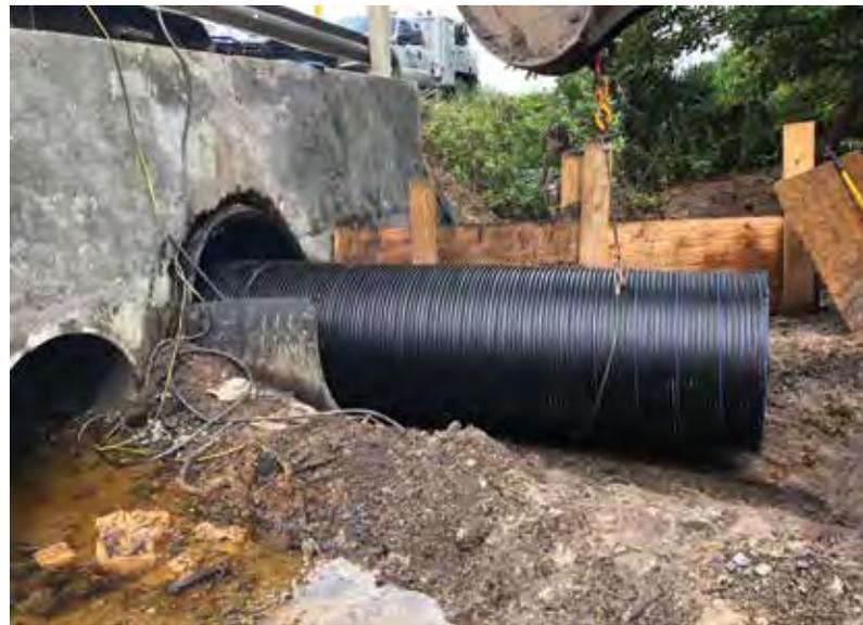
*The DuroMaxx SRPE Liner Pipe offered a fully structural relining solution*
