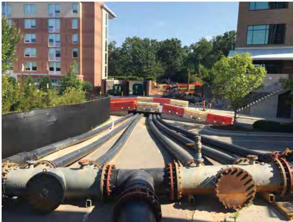
*Concrete Road Ramp with six 12-inch HDPE Bypass Lines*
