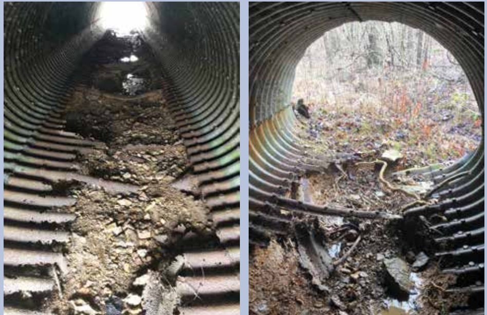
Pictures capture the deteriorated invert of the existing CMP culvert
