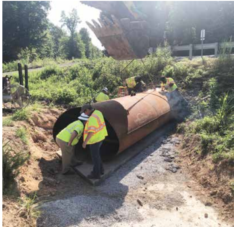
The liner section contained inverted bevels on the invert, allowing for welding to occur inside the liner. Welding of the top of the liner was accessible from the outside
