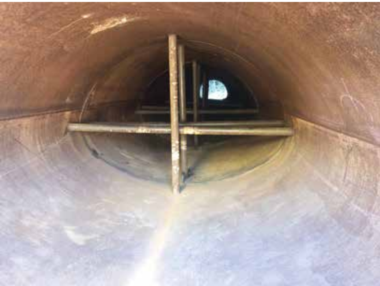
A look inside the InfraSteel liner, prior to bracing removal
