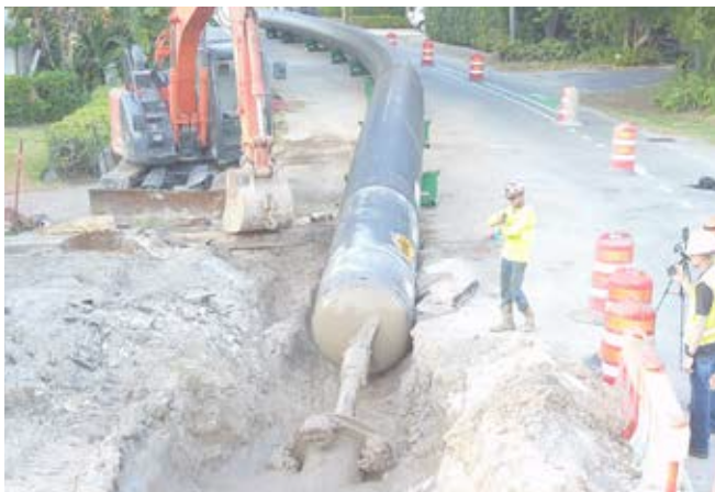
TDOT Maintenance crews cut and removed the deteriorated invert, and prepped the existing culvert for slip-line rehabilitation by pouring a concrete slab and laying channel iron for the InfraSteel liner to slide over
