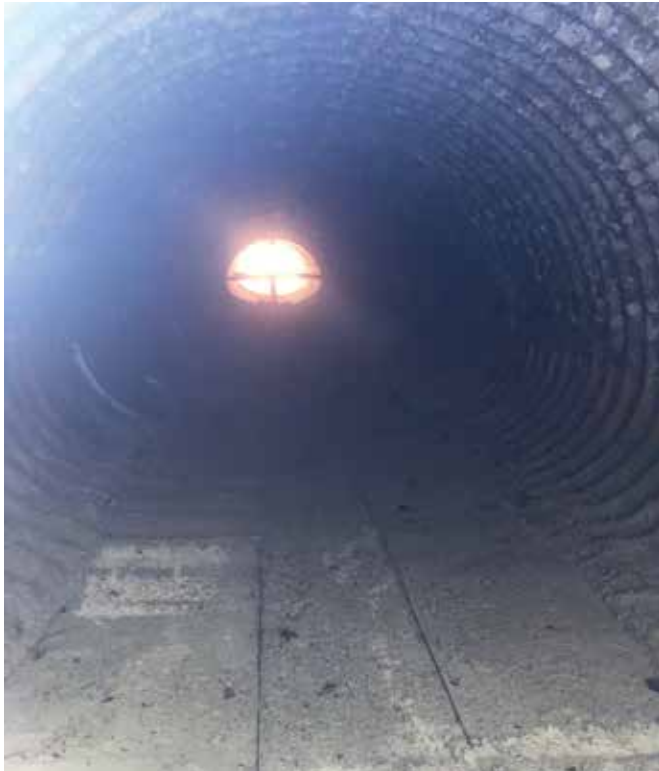
TDOT Maintenance crews cut and removed the deteriorated invert, and prepped the existing culvert for slip-line rehabilitation by pouring a concrete slab and laying channel iron for the InfraSteel liner to slide over
