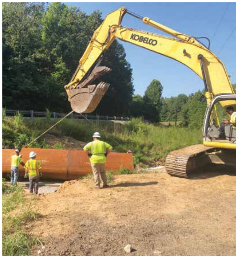
Liner sections being maneuvered into place, prior to slip-line insertion
