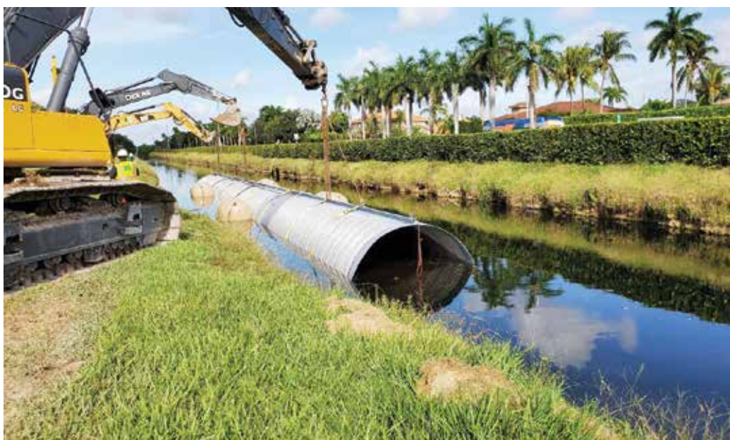
The liner pipe was installed under live flow using a unique anti-buoyancy method
