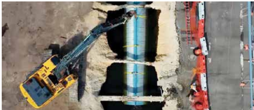
The HEL-COR liner pipe was installed with skid rails to ease installation
