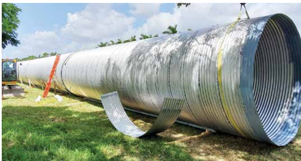
The 120-inch HEL-COR® ALT2 Liner Pipe was delivered directly to the site
