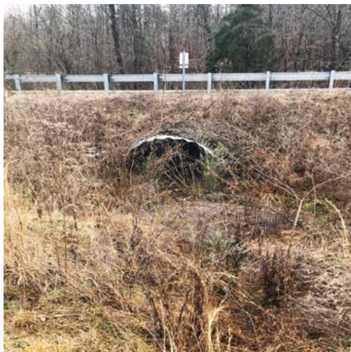
CMP Culvert located under SR-242. The structure was located under approximately 7ft of cover from the roadway and measured, 92" Span x 61.5" Rise x 64' Length
