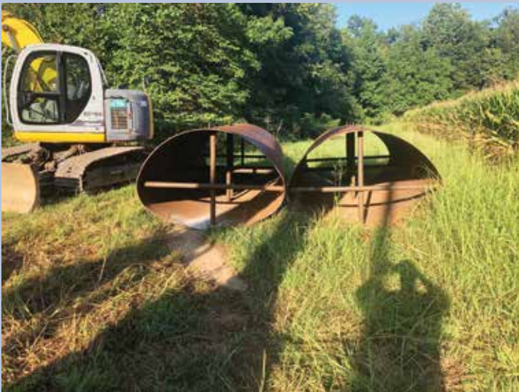
Liner sections on standby at the project site
