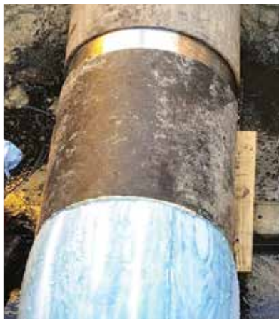
Figure 3. End termination of a 24-inch Force Main in South Carolina
