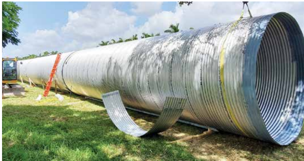
The 120-inch HEL-COR® ALT2 Liner Pipe was delivered directly to the site
