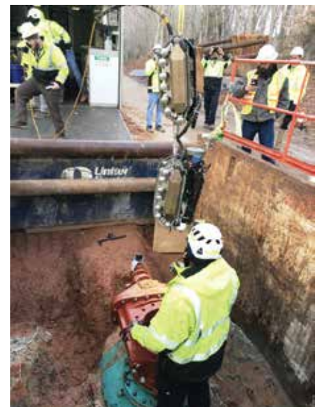
Robotic Crawler Insertion in 36-inch PCCP
