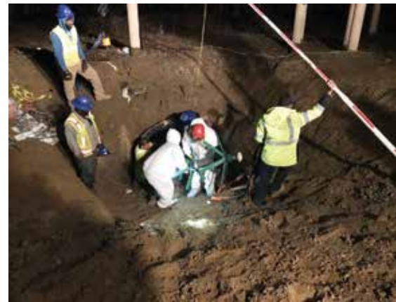
Extraction of PipeDiver Following Inspection of Lake Crossing D
