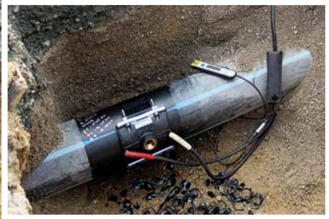
Typical Electrofusion Joint
