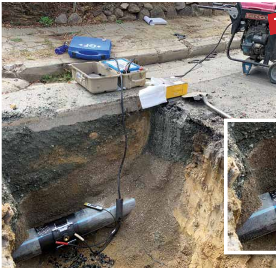
Typical Electrofusion Joint
