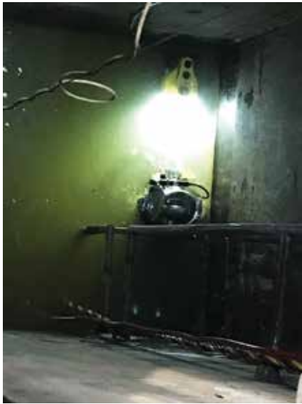
Diver Assistance with Robotics Inspection of 72-inch Intake
