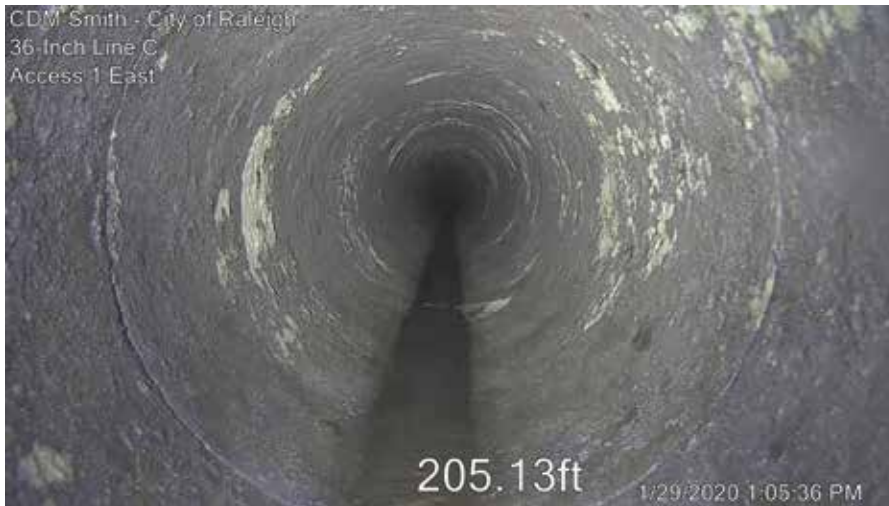
36-inch PCCP Inspection with Robotics
