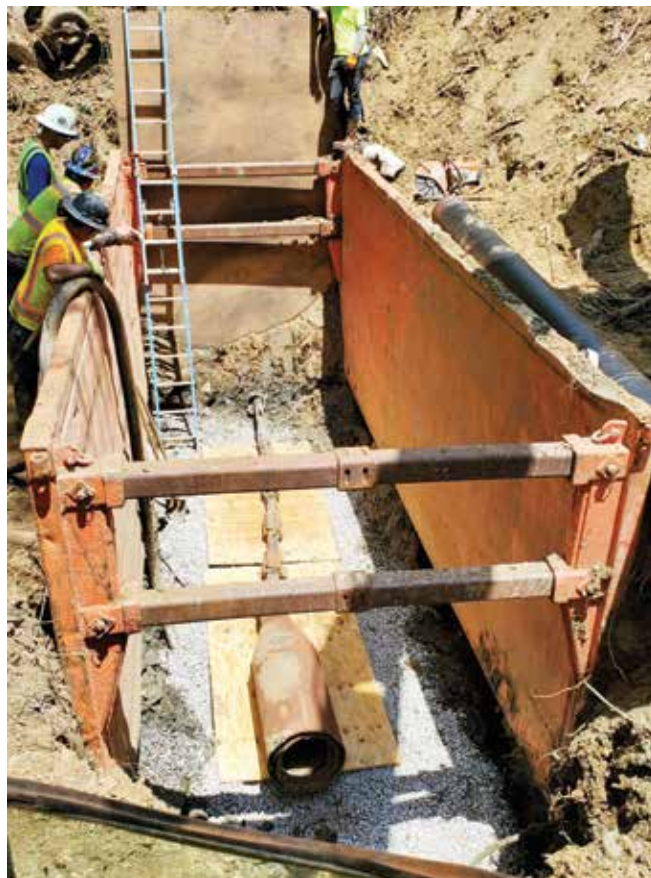
Bursting ductile iron pipe has become more prevalent with static pipe bursting systems. Special bladed rollers are needed to properly split the difficult pipe material
