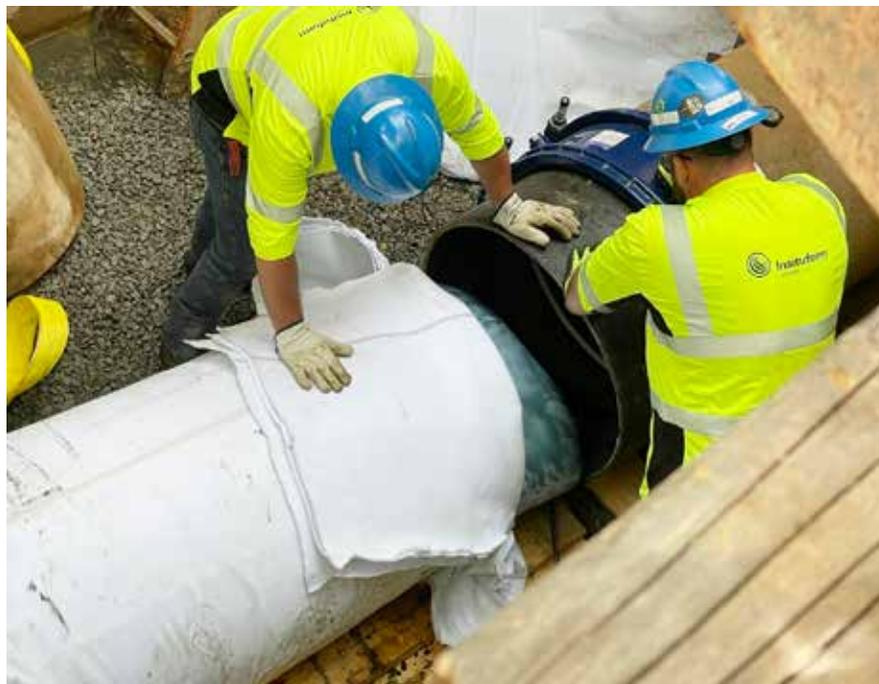
*Using an updated methodology, termination of the liner was done outside of the host pipe*
