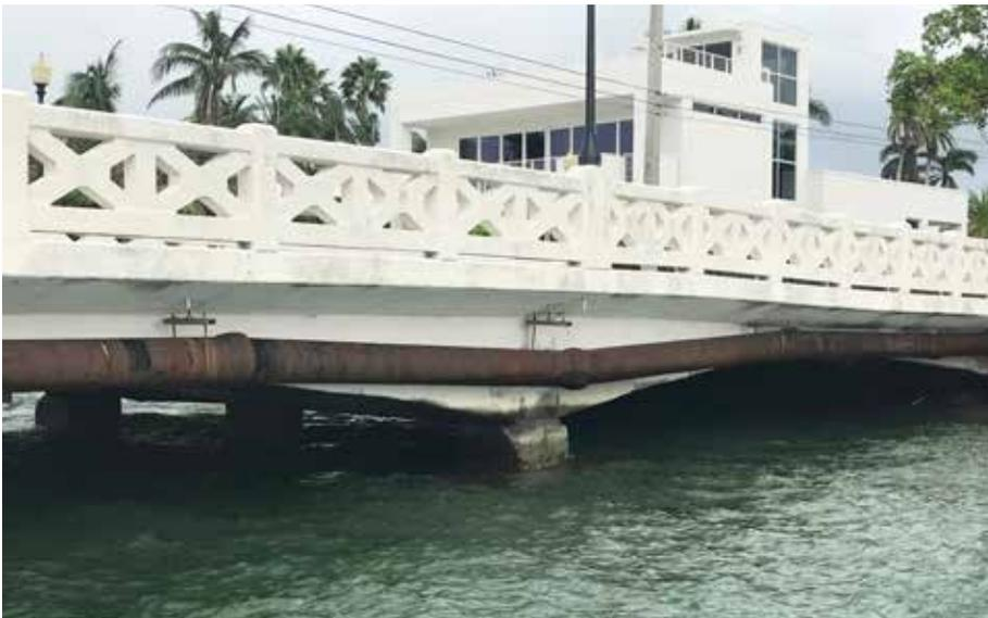
Existing water main aerial crossing showing significant joint deflection, pipe corrosion, and pipe support failures
