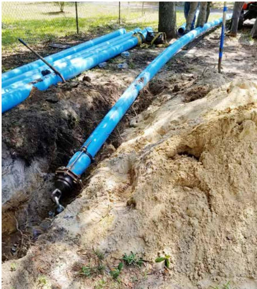
*A fire protection line is designed with a larger diameter pipe*
