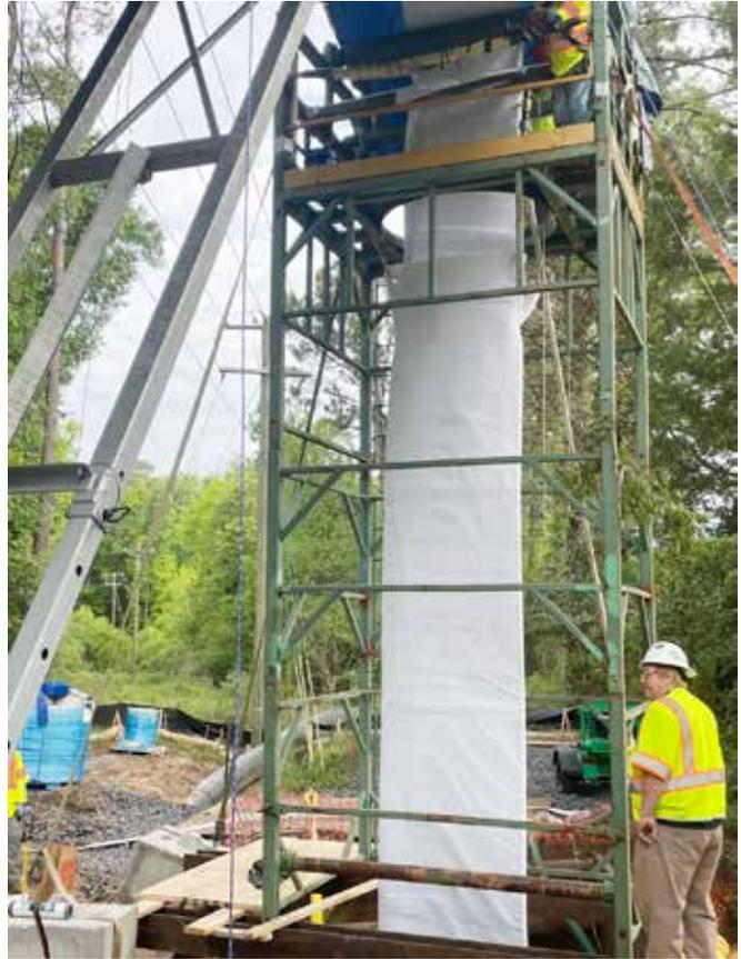
*Historically, installations of extremely long lengths and larger diameters are accomplished with the “Over-the-Hole” method*
