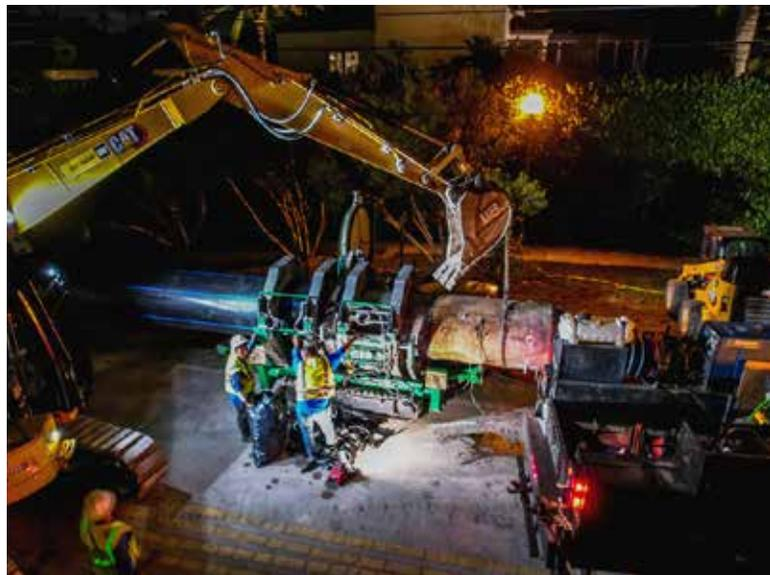
*Butt fusion of the pulling head onto 36-inch HDPE piping*
