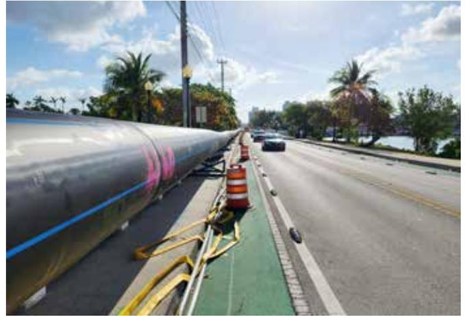
MOT plans allowed for flagged two-way traffic when pipe was fused and strung out for pullback along the two-lane road
