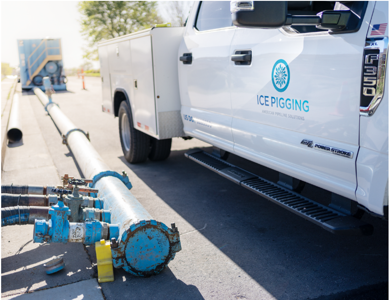
Ice Pigging is a minimally invasive technology with small surface footprint
