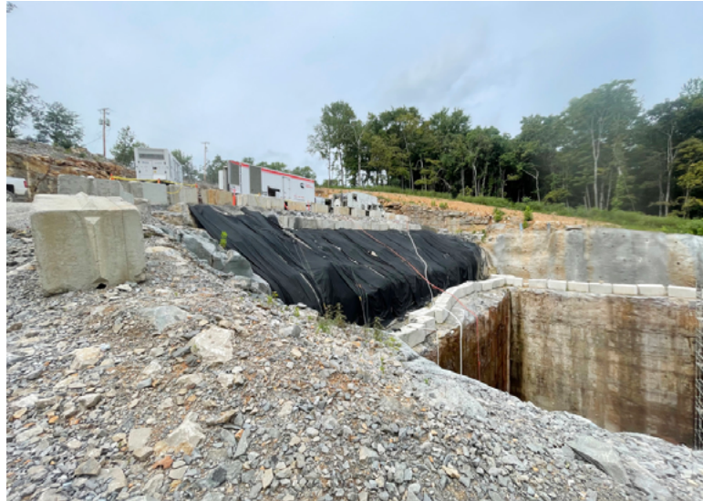
An 80-foot deep jacking shaft was sunk behind the river bluff
