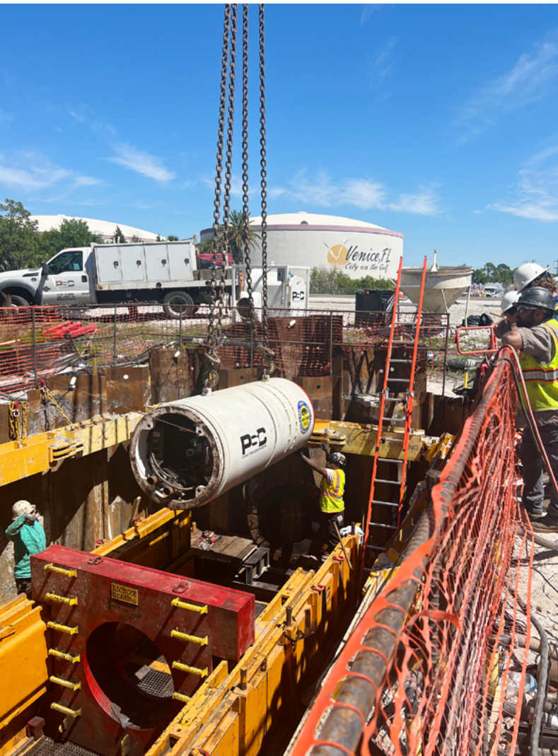
Microtunnel launch shaft
