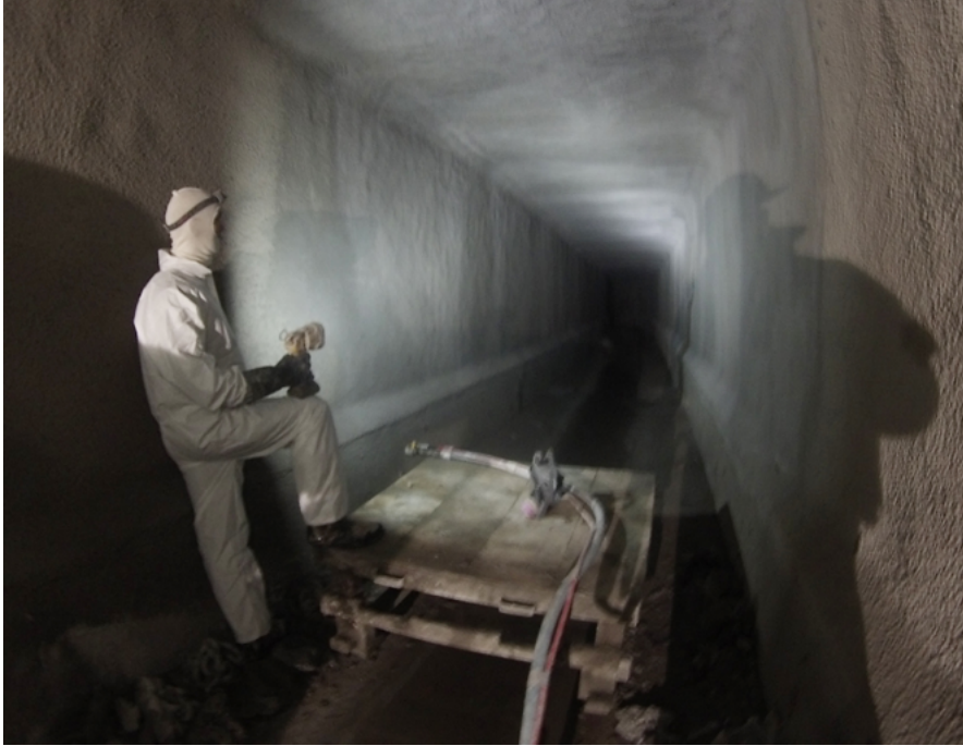
Figure 3. Geopolymer SAPL provides a true structural rehabilitation
