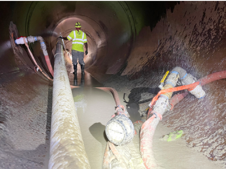
Three 4-inch sacrificial grout lines were installed in the casing
