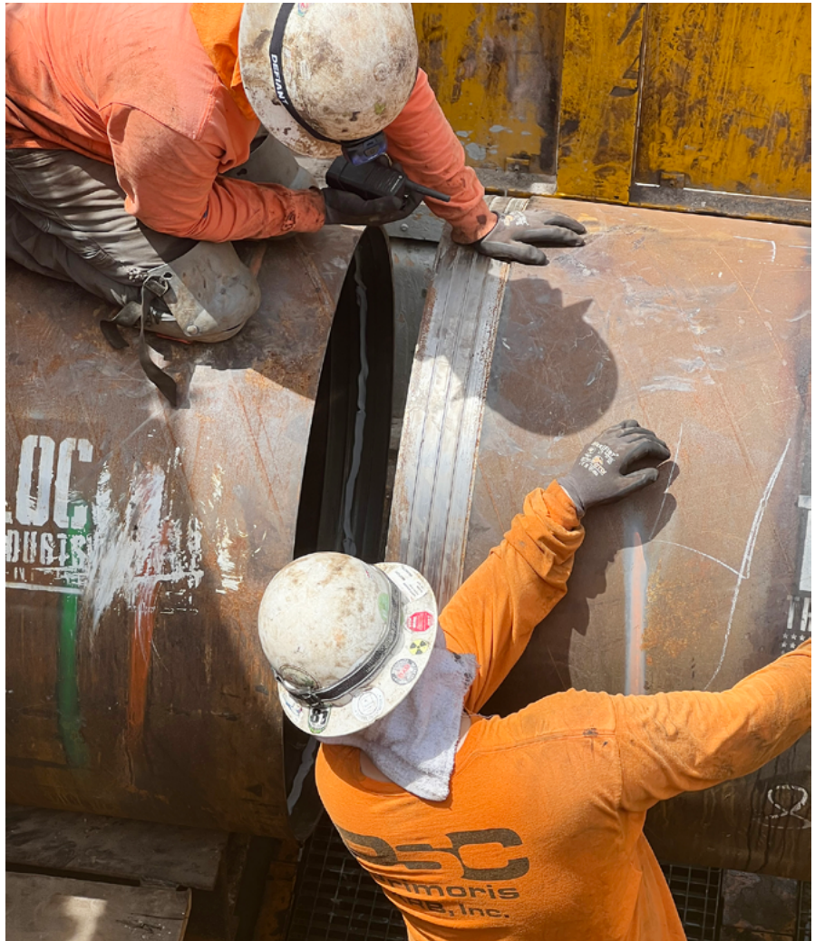
Vadnais personnel line up the Tri-Loc steel pipe
