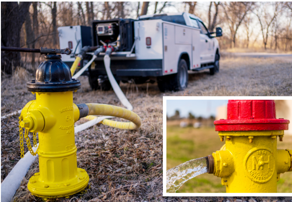
Ice Pigging process utilizes existing fittings such as hydrants
