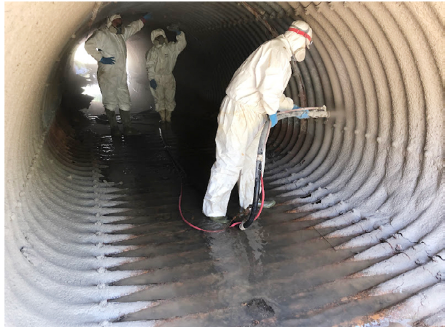
Figure 2. Geopolymer is used as a SAPL either by hand spraying or spin casting
