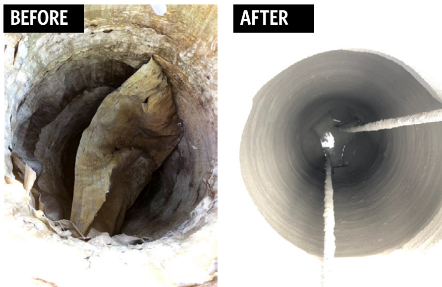
Figure 6. Geopolymer is becoming the preferred application for manhole rehabilitation due to its versatility and resistance to corrosion
