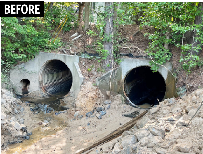
Figure 4. Twin 60-inch CMPs were rehabilitated with minimal neighbourhood impact and no road closures
