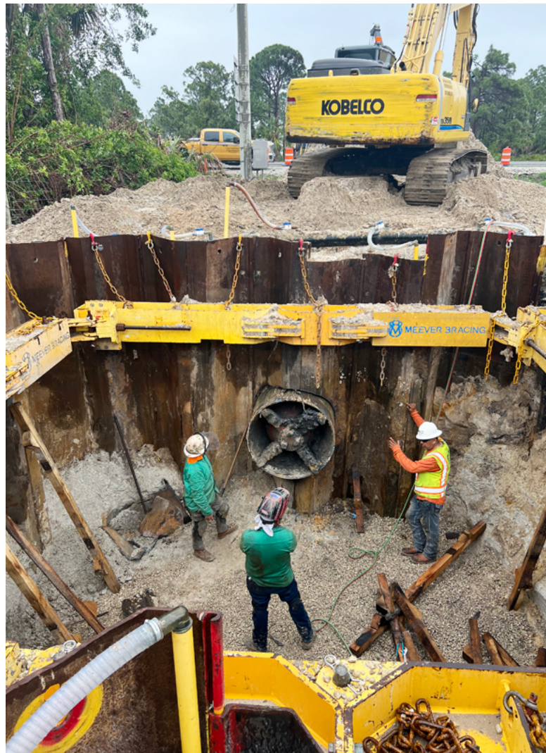
Breakthrough of the 42-inch microtunnel machine into the reception shaft
