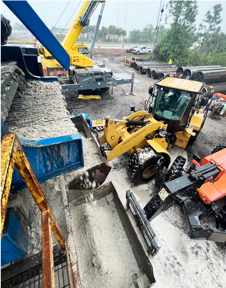
Excavated spoils being removed by the two-stage slurry separation plant
